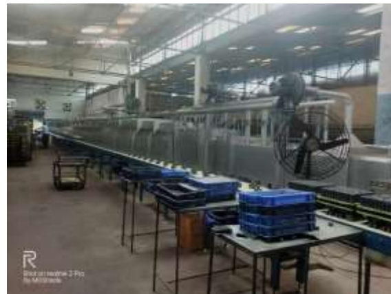
Furnace for sintering of the soft magnetic cores (Dry process)
